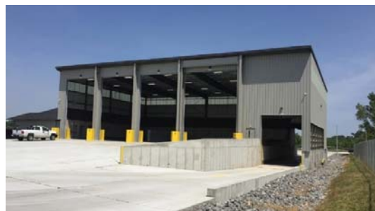
Figure 2: Typical waste transfer station. Source: The Cape Girardeau Transfer Station in Montana, designed and built by Cambridge Companies.
