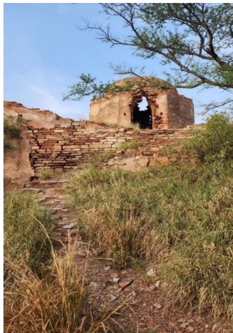
Figure 6 Temple atop the Fort
