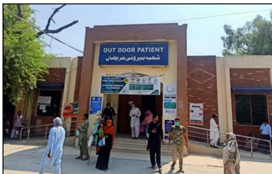
Figure 20 Too steep ramps and wrong parking at main entrance of OPD
