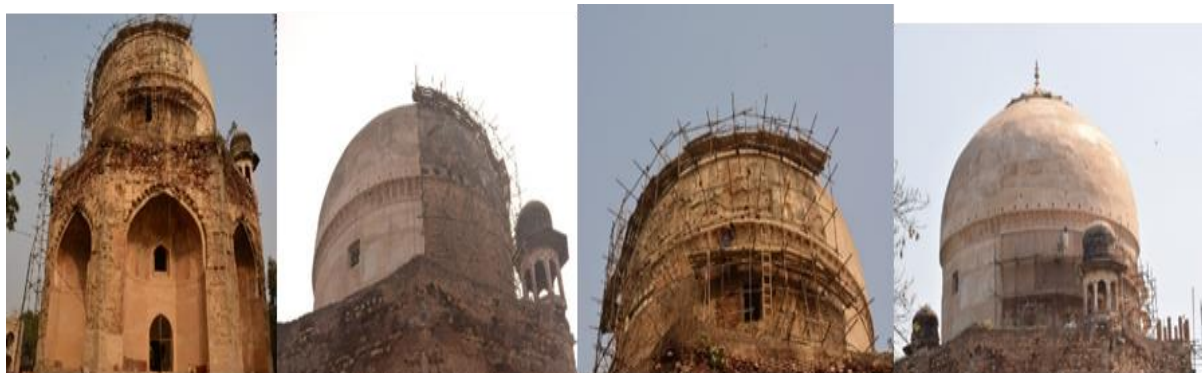
Figure 5: Image showing the conservation works of Dome and its cylinder.
