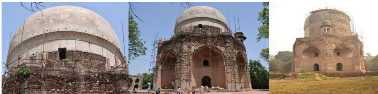
Figure 6: Images showing the repair work of the facades and peshtaq with arched openings.
